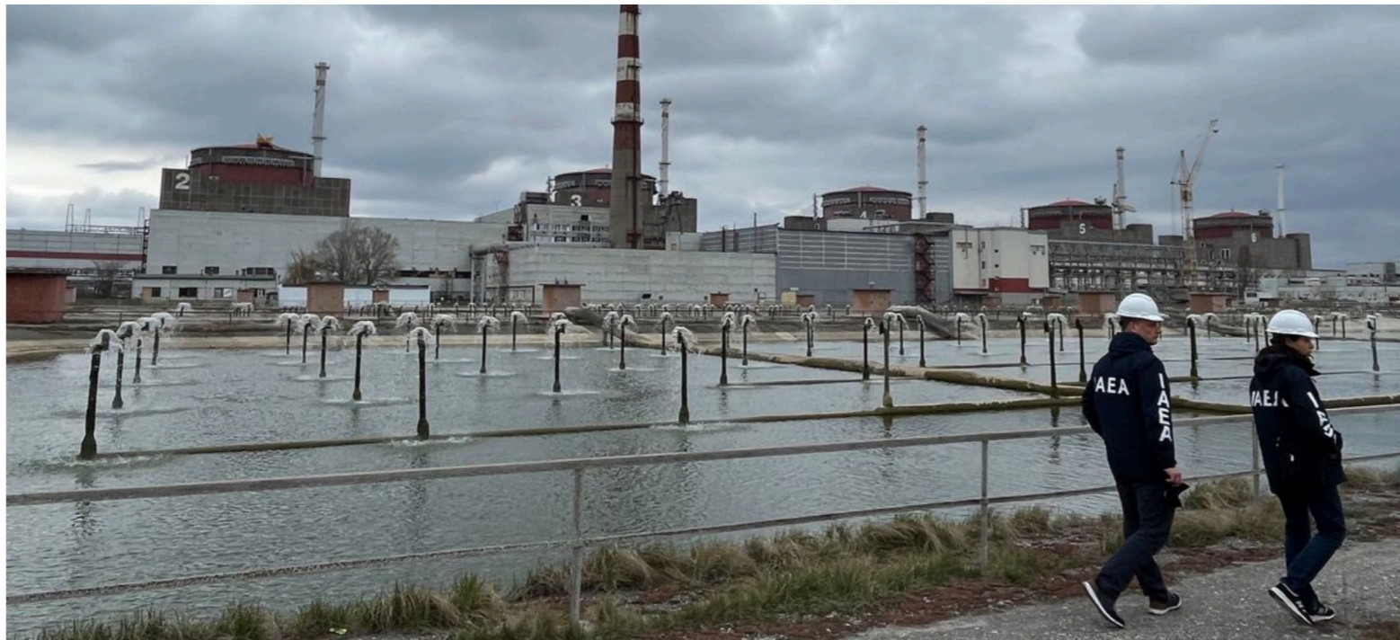
© IAEA/Fredrik Dahl | An IAEA expert mission team walks around the Zaporizhzhya Nuclear Power Plant and its surrounding area. (file)
